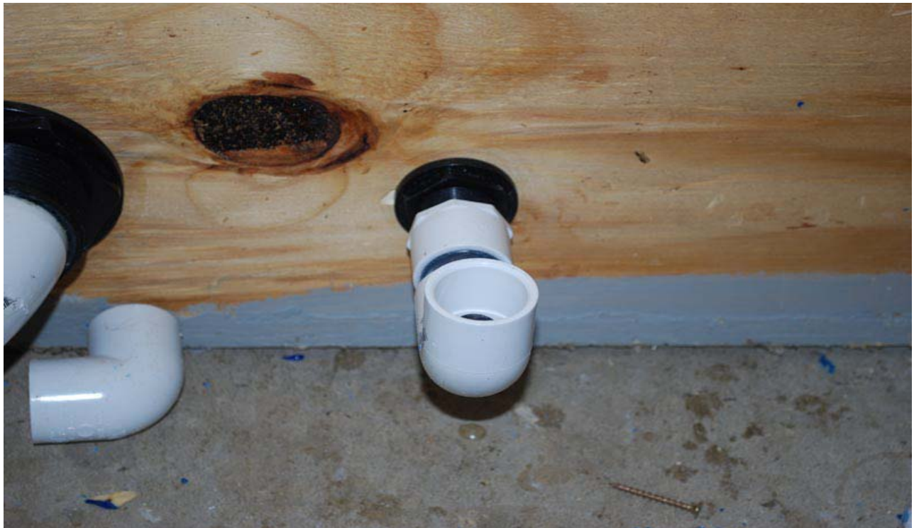
Building the sight glass for water level.
